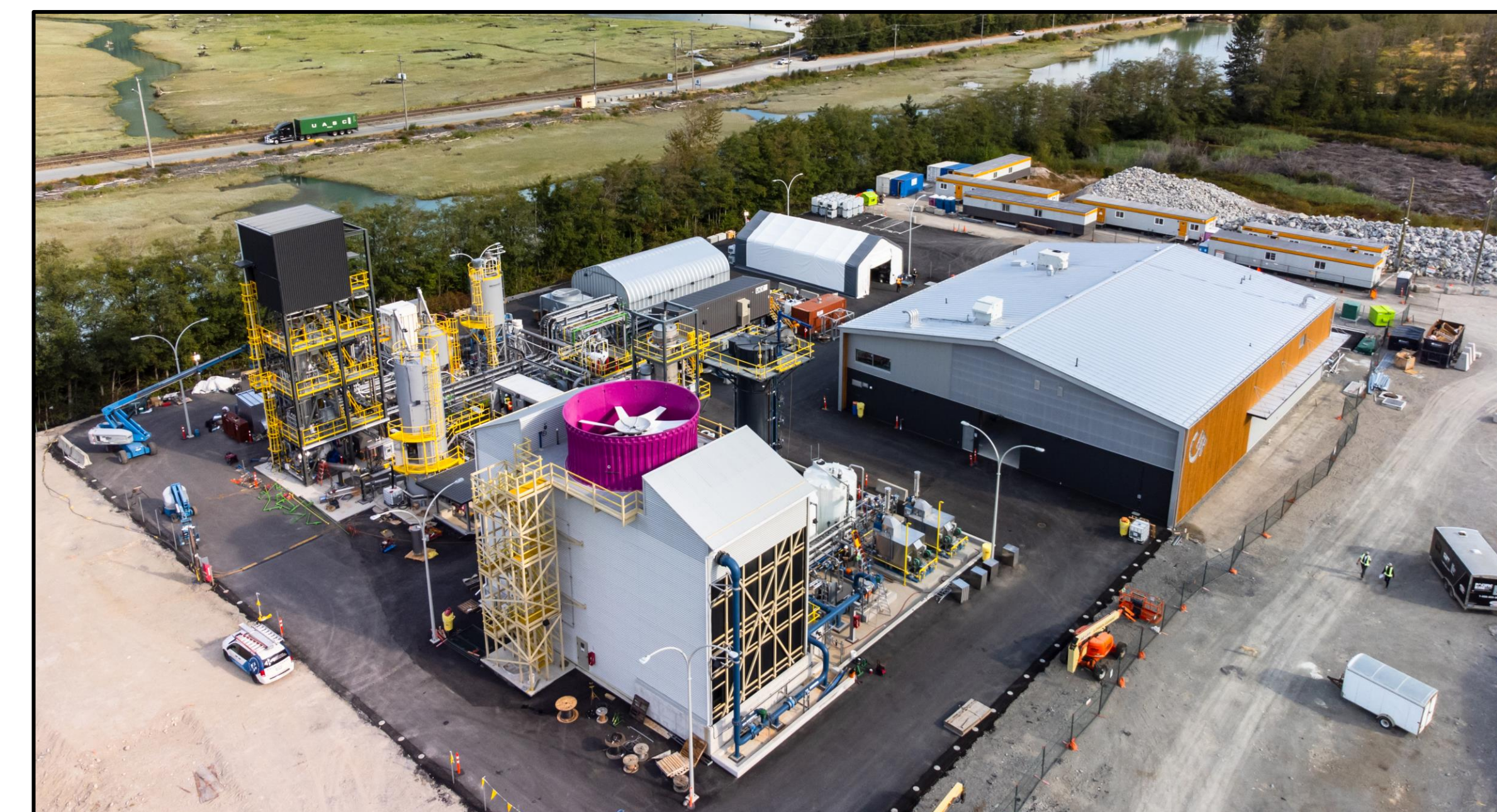
The Carbon Engineering Innovation Centre is a DAC demonstration facility used to perform research and development on CE's technology
